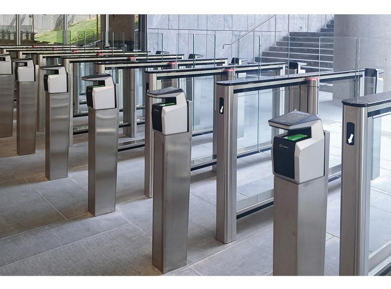
Speed gates are supplemented with stands for 3D scanners to support biometric fingerprint access.
